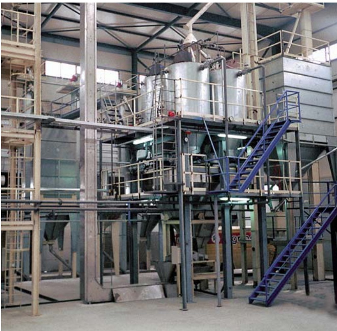
1 - 2 t/h parboiling plant
